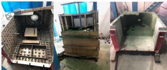
Fig. 3. Building Process of The Side Chamber Refractories.
