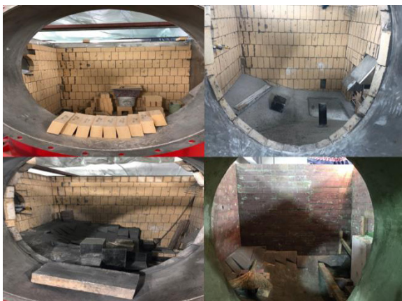
Fig. 4. Building Process of The Body Refractories.
