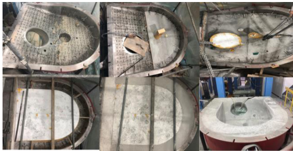
Fig. 2. Building Process of The Lid Refractories.
