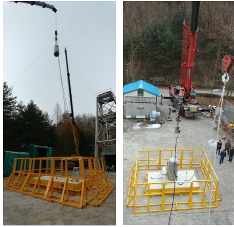
Fig. 3. Preparation for drop test.
