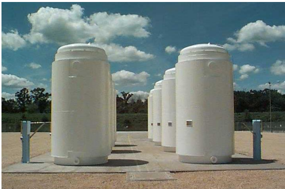
Fig. 4. Transportable dry storage casks.
