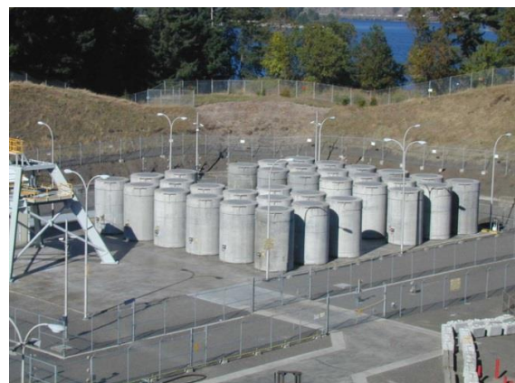
Fig. 1. SNF dry storage facility.
