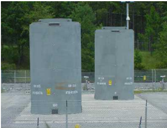
Fig. 3. Canister-based dry storage casks.
