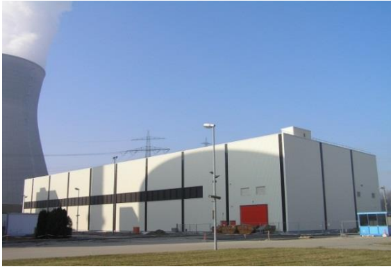
Fig. 2. SNF dry storage building.
