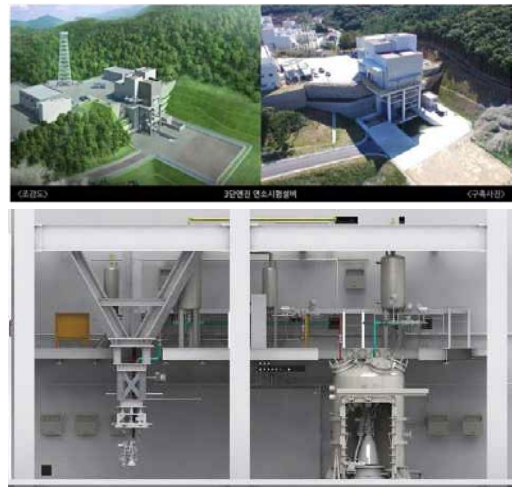
Fig. 2 Upper stage engine test facility
