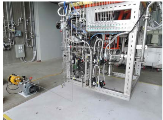
Fig. 4 Vacuuming of ignitor line
