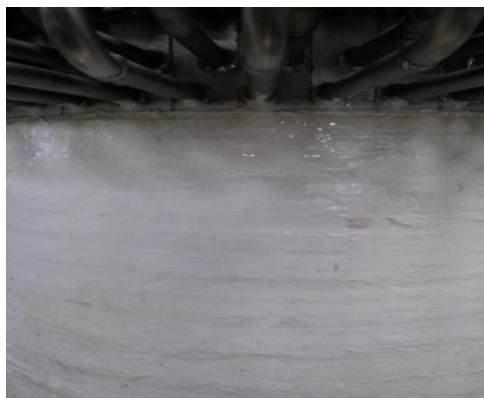
Fig. 1. Photo of external wall coating material of CCIM.
