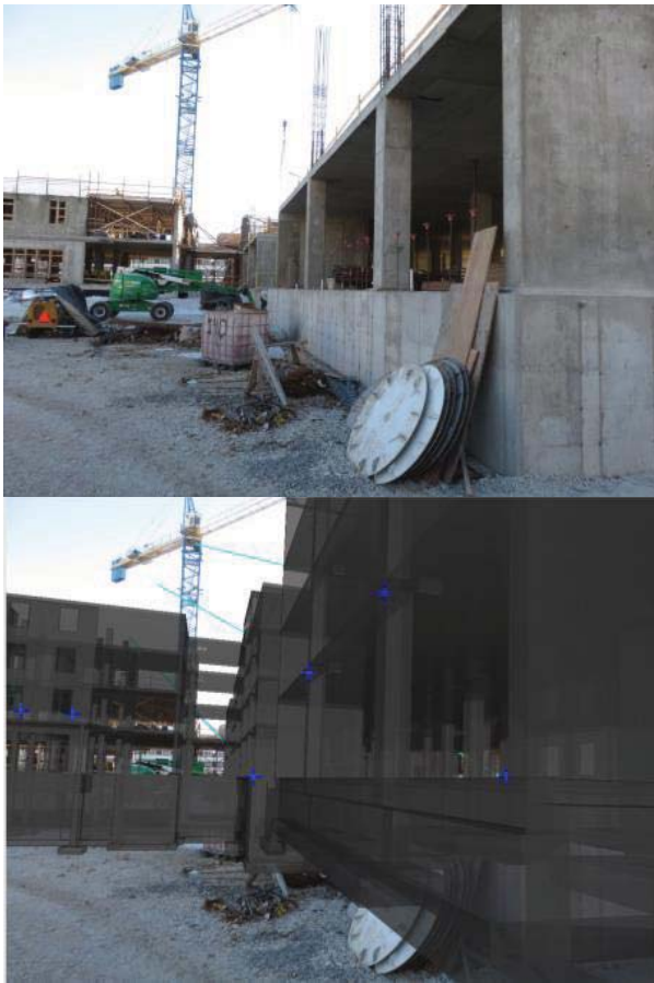
Fig. 4. An image registered with a BIM by BIM-assisted SfM.
