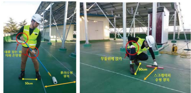
FIGURE I. PRIMER PAINTING (L) AND POLYURETHANE PAINTING (R)
