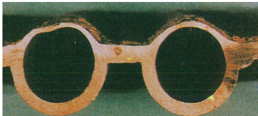
Fig. 1 Water wall tube corrosion [2]
