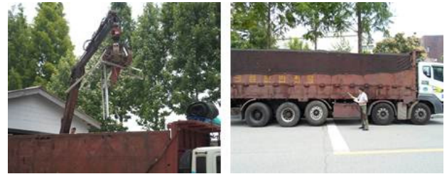
Fig. 4. Metal radwastes loaded on a truck (left) and direct contamination measurement (right).
