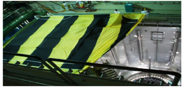
Fig. 3. Covering the reactor pool against airborne activity(Germany).
