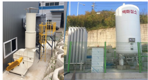
Fig. 2. Copper dust collector(left) and N2 carrier gas supply system(right).
