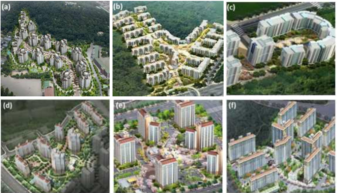
Figure 1. Bird's-eye views for each apartment complex: (a) Site 1, (b) Site 2, (c) Site 3, (d) Site 4, (e) Site 5, (f) Site 6
