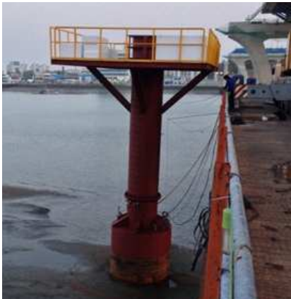
Figure 1 Suction pile prototype in test site.
