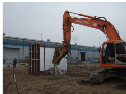
(a) After installation
