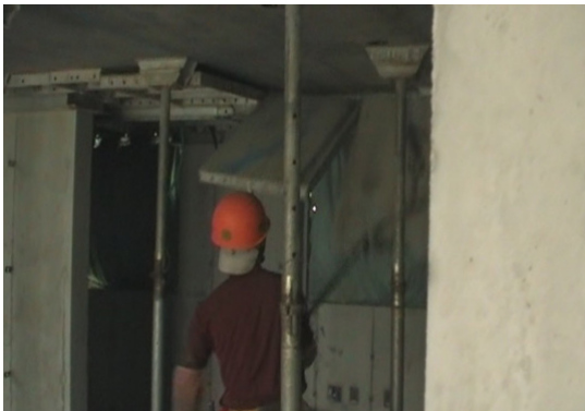
Figure 6 Demolition of gangform at construction site
