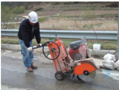
(a) Before installation
