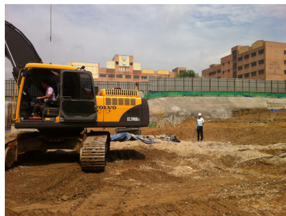
(a) Before installation
