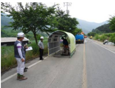
(b) After installation
