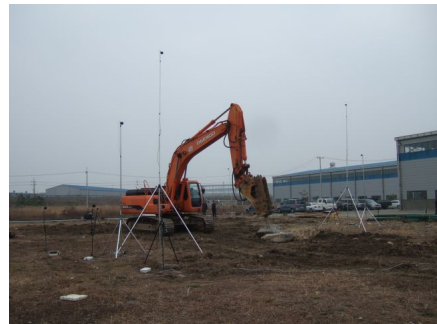
(a) Before installation
