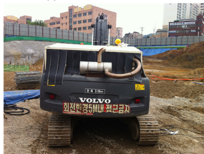
(b) After installation
