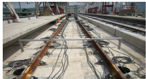
(a) Slab lifting(Multi channel hydraulic pressure jack-up system)
