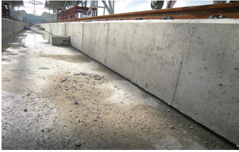
(b) Slab lifting and track status Fig. 4 Test construction process
