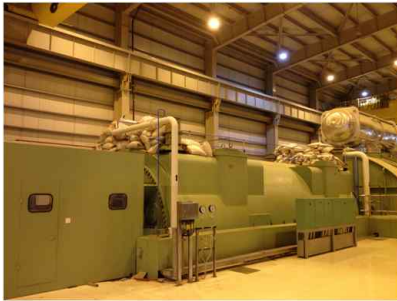
Fig. 2 The loading of lug and sand bag on the generator stator
