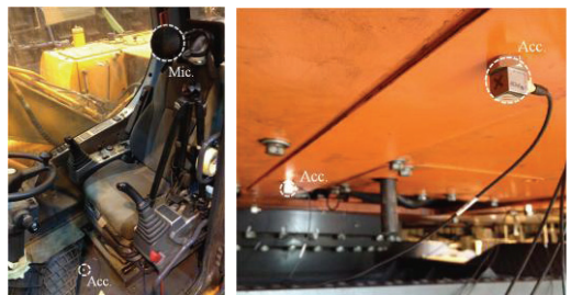
Figure 2 Measurements of operational noise and vibration for the cabin and for indicators
