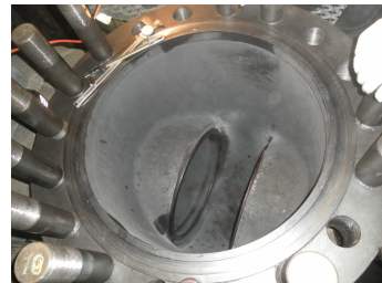
Fig. 1 View on seat ring of isolation valve
