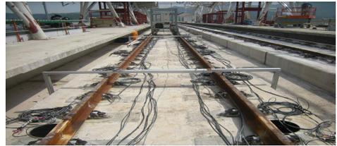
(a) Slab lifting(Multi channel hydraulic pressure jack-up system)
