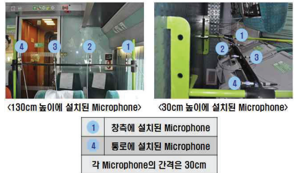
Fig. 2 Microphone installation place
