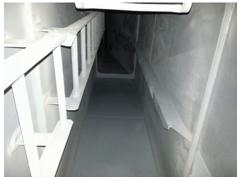
Fig. 4 Hull duct inside (upward)
