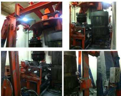
Fig. 1 Details of zinc flake coating room
