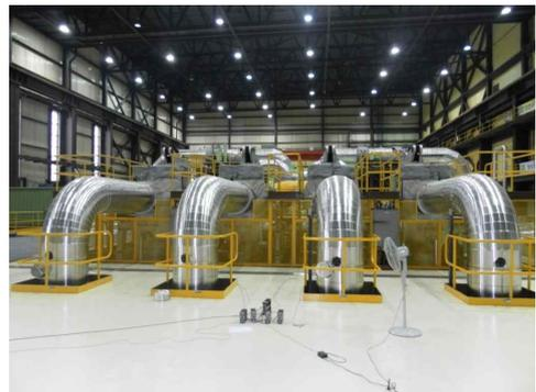
Fig. 2 26" Pipe Lines before chest valves
