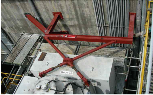
Fig 11 a stiffener during installing
