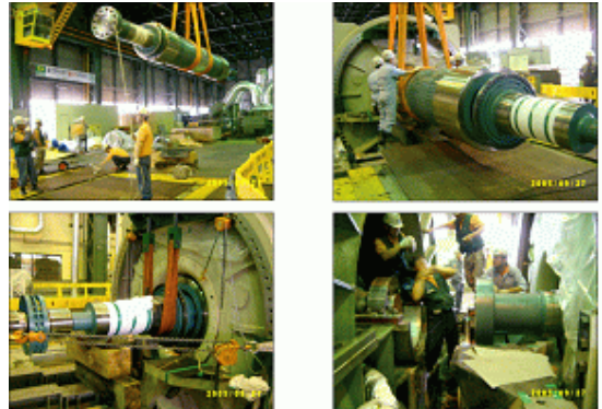
Fig. 6 Installation of new generator
