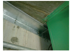
(c) After installation
