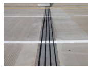
(c) Rail joint
