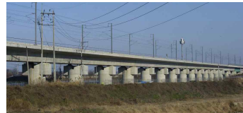
Fig 1. View of Seongdong Viaduct
