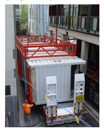
Factors identified by Blismas (ed.) included site access and space to manoeuvre, availability and access for cranage, high winds and available hook time. Factors encountered by UB included power lines and other services on-site or on route, road width, bridges and turning circles available for delivery, Council restrictions on CBD access during business hours and cranage. Subsequently the project required permanent installation of a Tower Crane in an adjacent car-park.
