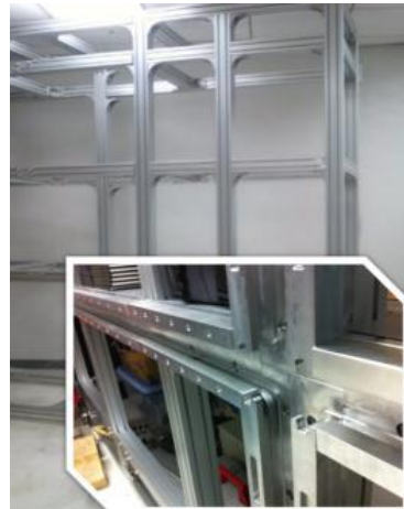
Fig.1 Mock-up building with Built-in Guide Rail
