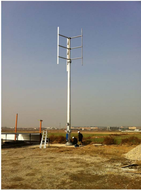
Fig. 17 Final assembly of 6 kW class VAWT model
