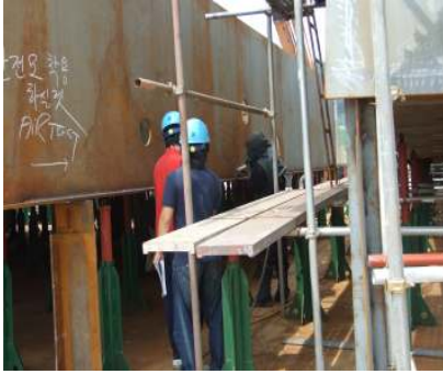
Photo. 1 A Scene of grinding work
