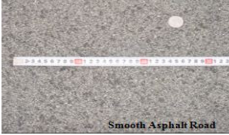
Fig. 8 Smooth Asphalt Road
