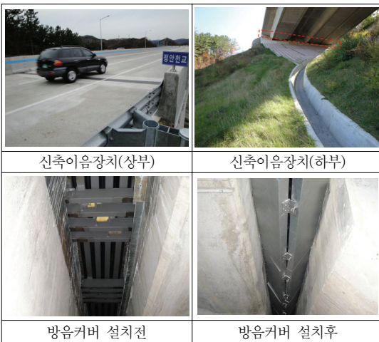
Figure 1. Photos of rail-type bridge joint and noise cover
