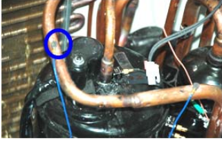
Fig. 3 Measurement of acceleration at pipe
