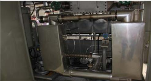
Fig. 2. Catalytic system for disposition of organic radwaste solution
