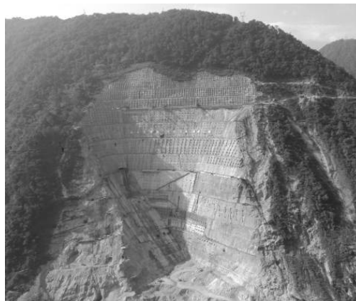
Fig.1 The right bank slope after excavation of the dam
