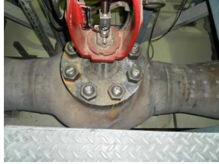
(a) Clamp of damaged steam
