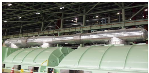
Fig. 1 LP turbine casing
