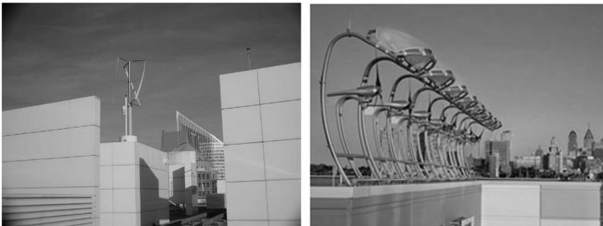
Fig. 1. Building integrated wind turbines(left: vertical, right: horizontal axis type wind turbine).
