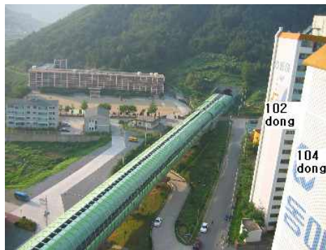
Photo. 1 The scene of sound absorption tunnel on the elevated railway
