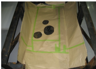
Fig. 13 Inspection of leakage
