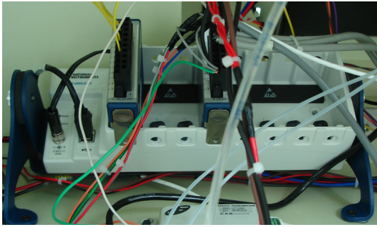
Fig. 5 Data Acquisition System
