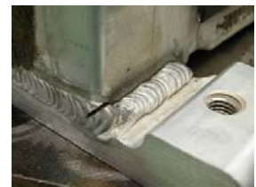
(b) Failure mode
