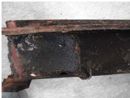
Fig. 1 Corrosion of Under-Frame
