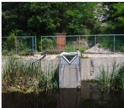
Fig. 2. V-notch Weir
