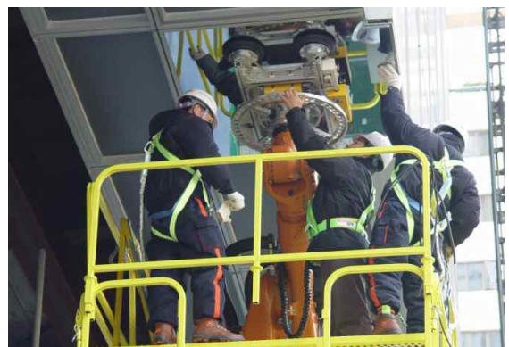
Fig. 2 Ceiling glass installation robot
