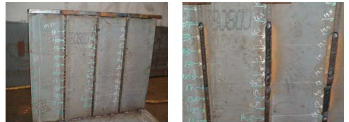
Fig. 7 Welding result using automatic welding robot
