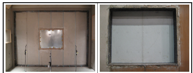
Fig 1. Installation of specimen
