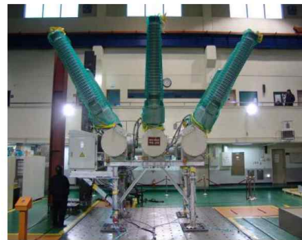
Photo. 1: Support-mounted configuration of 245kV GCB on shake-table
